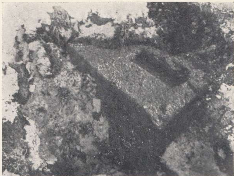
Fig. 4. STONE WITH SOCKET TO TAKE BEARING OF WATER-WHEEL, YELLOWMEAD.
